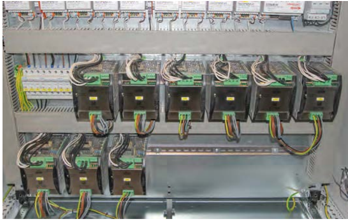
Emparro power supplies in the control cabinet
